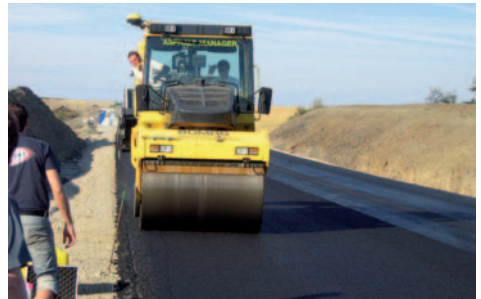
Fig. 88 BW 174 AM with BCM 05 and GPS
