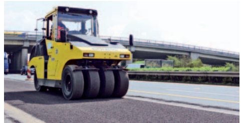
Fig. 62 Initial compaction, pneumatic tired roller BW 24 RH
