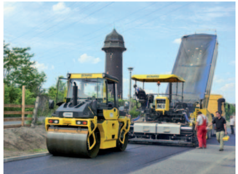
Fig. 58 BW 154 AP compacting a wearing course with a curbstone
