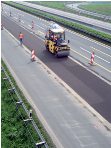
Fig. 70 Compacting a longitudinal joint
