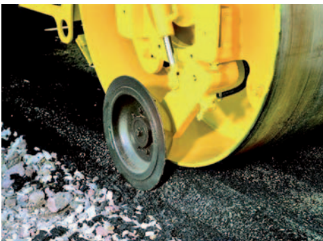
Fig. 39 The compressing roller produces a slanted and smooth layer edge
