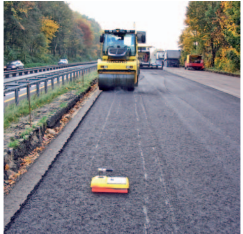
Fig. 83 Compaction measurement for comparison with E_{ViB}
